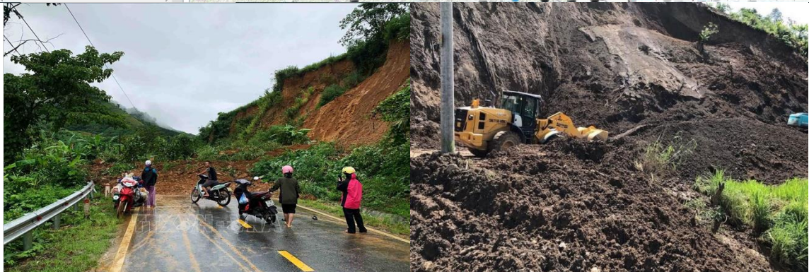
Figure 1.4. Landslide occurrence at Muong Te district, Lai Chau province as a result of 3hr-accumulated rainfall > 100mm
